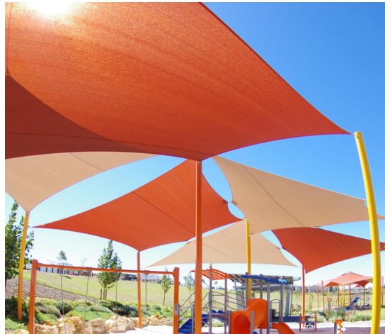
SHADE & TENSILE STRUCTURES
