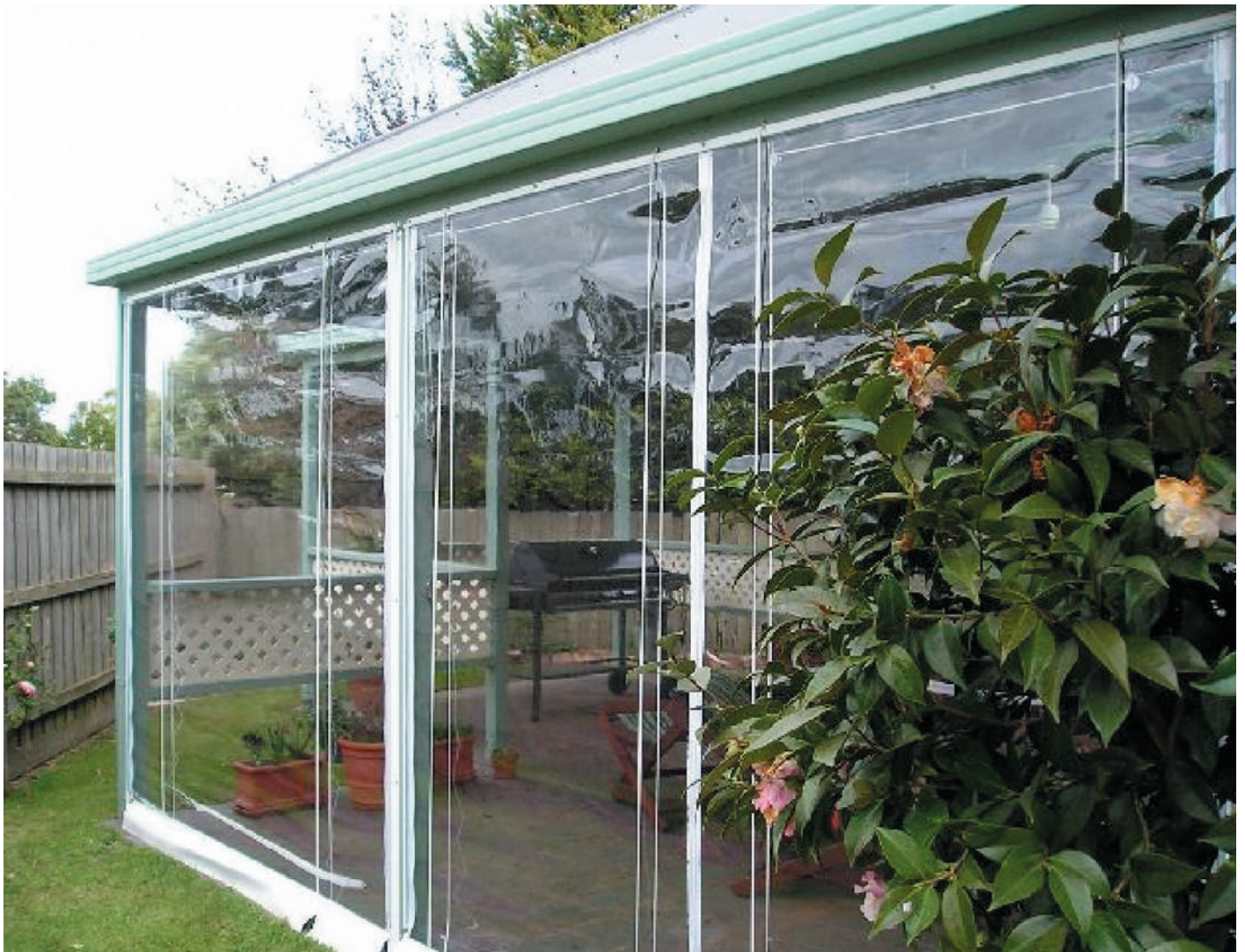
■ Figure Twelve – Drop-down blind operated using a cord and pulley system, which has been largely superseded by crank or guided systems.
