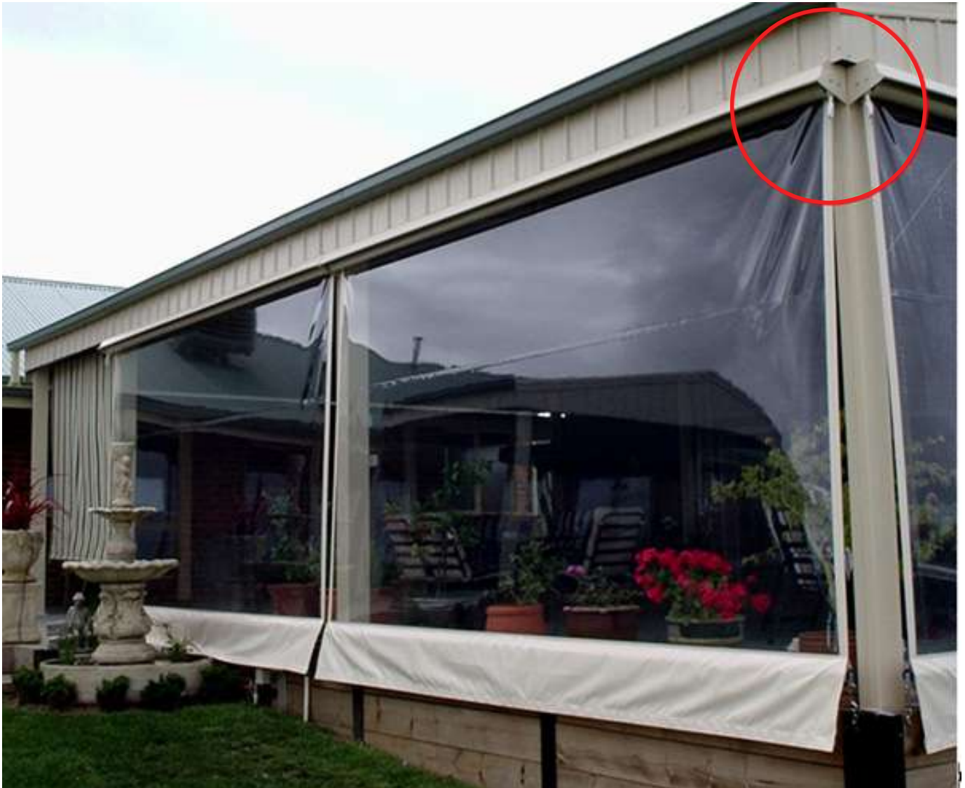
■ Figure Thirteen - An example of a crank operated straight drop blind, manufactured from clear PVC. The crank hook is circled (Photo courtesy of C.E. Bartlett)
