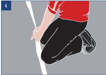
Measure and cut the second piece from the roll. Position the second piece with the edge overlapping the first by approximately 5cm and mark a guide line on the floor with a pencil at the next seaming edge. For ribbed carpets, ensure the ribs are aligned on both layers.
