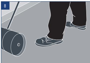
When the floor has been completely covered, re-roll the area again to maintain good adhesive contact.
